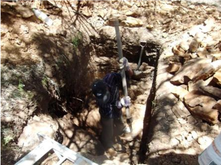
Septic tank dug by hand took 3 days digging ( thru rock too)
