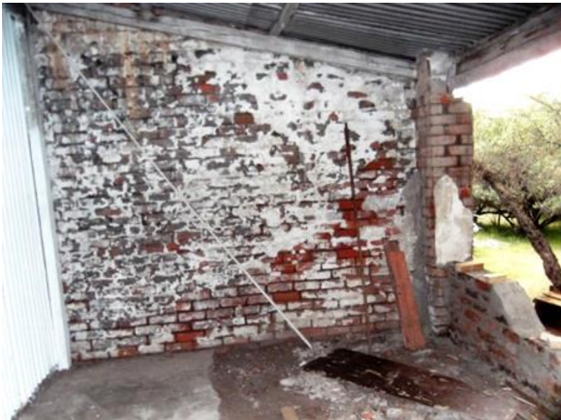
Walls and floor on the verandah need rebuilding and plastering
