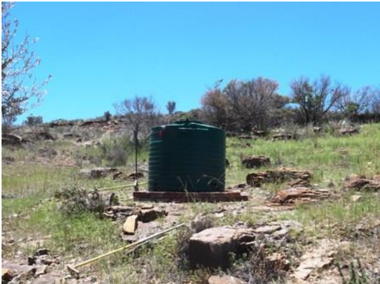
We have installed a tank for a water supply. Now we have a toilet and a sink with running water, but it is not drinkable water.
